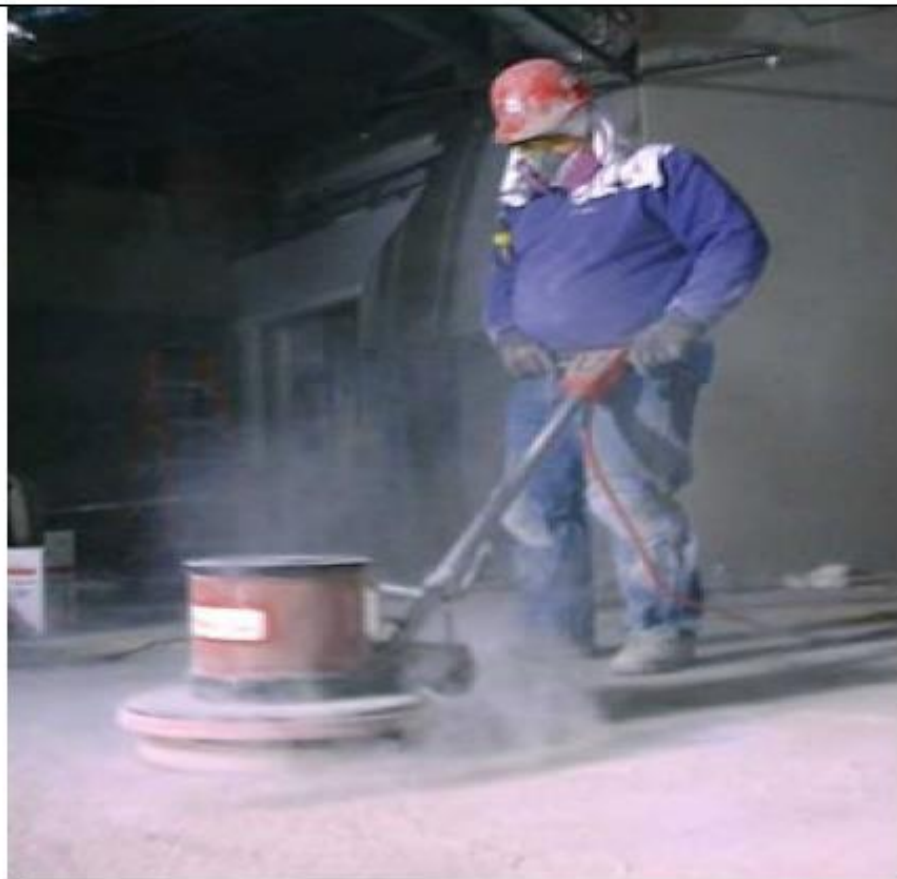
Poor Practice – sanding concrete floors without on-tool extraction (GDWW, B)
