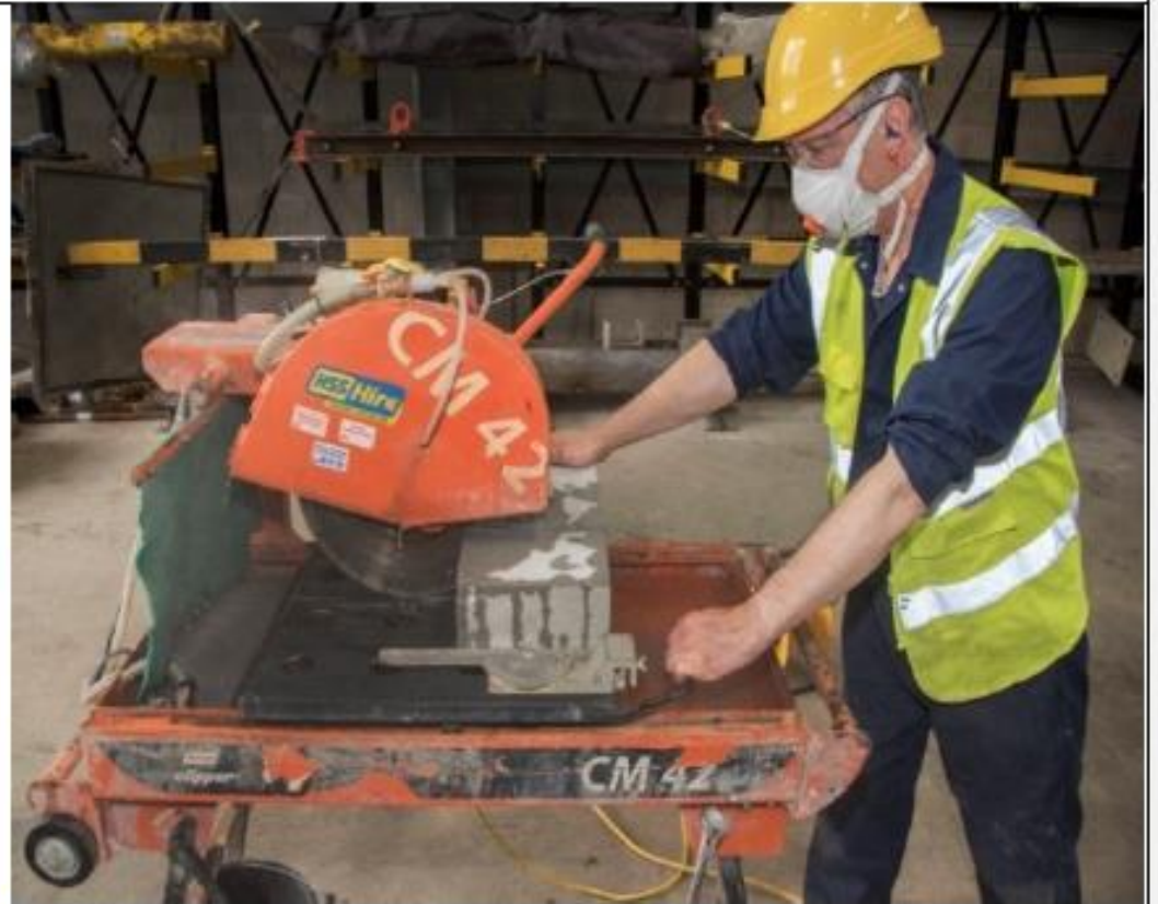
Good practice – Use of water suppression (shown) and RPE worn by the operator (HSE, GB)
