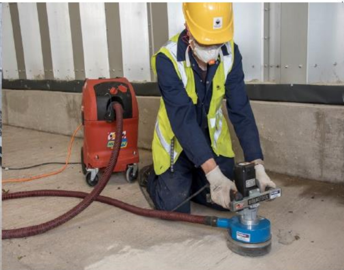
Good practice – Using a hand-held grinder with on-tool extraction (HSE, GB)
