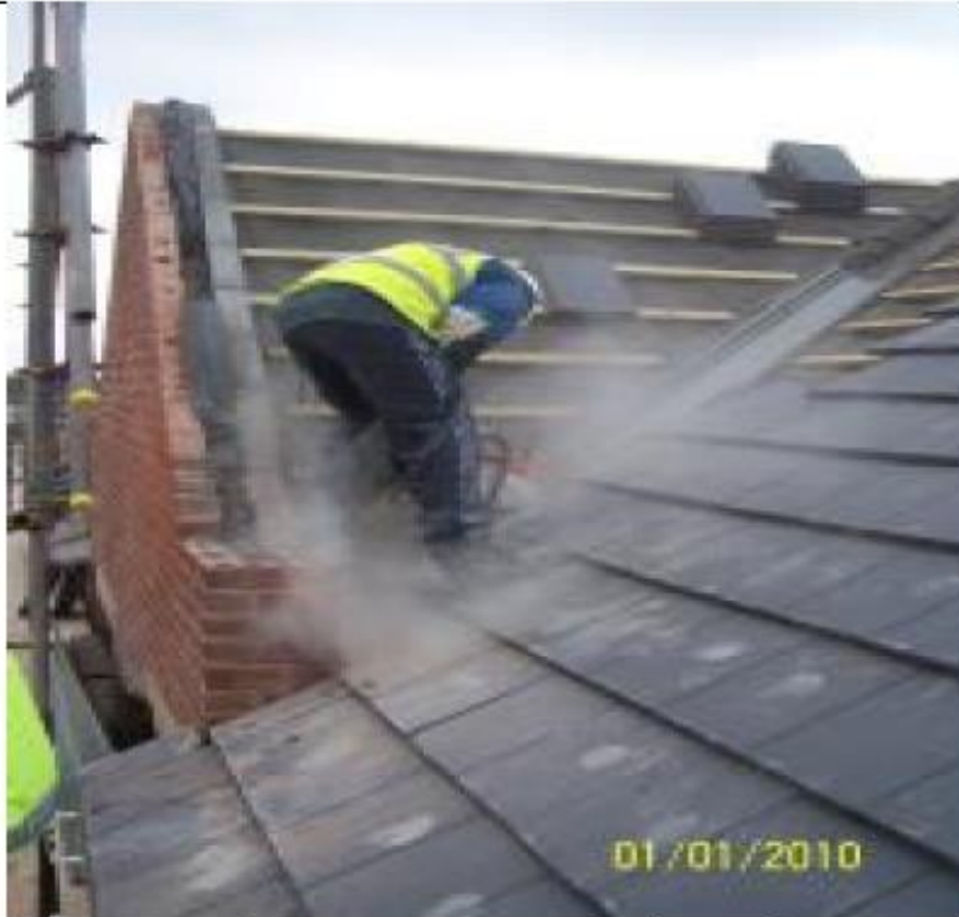
Poor Practice – Cutting roof tiles without control measures (National Federation of Roofing Contractors Ltd, GB)
