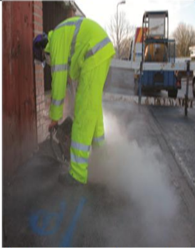
Poor practice – no dust suppression or RPE (HSE, GB)
