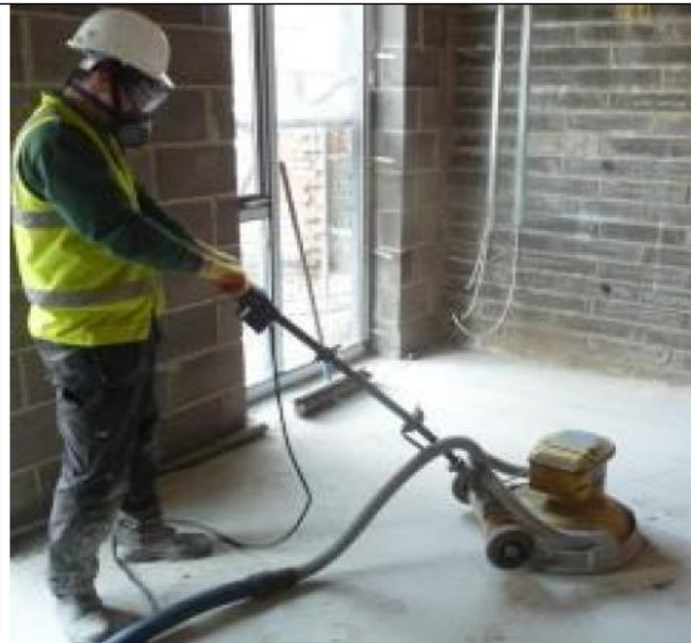
Good practice – sanding concrete floors with on-tool extraction (HSE, GB)
