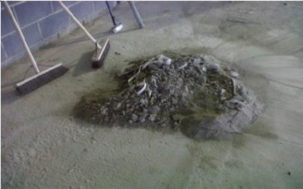
Poor Practice – Removal of rubble using dry sweeping (HSE, GB)
