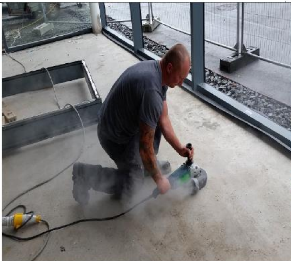
Poor Practice – Using a hand-held scabbler without on tool extraction (David Flynn Ltd, IE)
