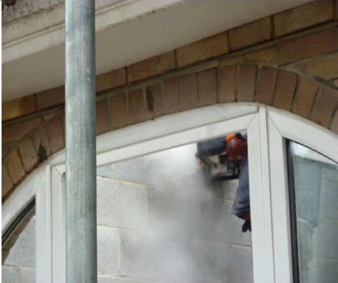
Poor Practice – Chasing concrete with no on-tool extraction or RPE (Safer Sites Website, GB)
