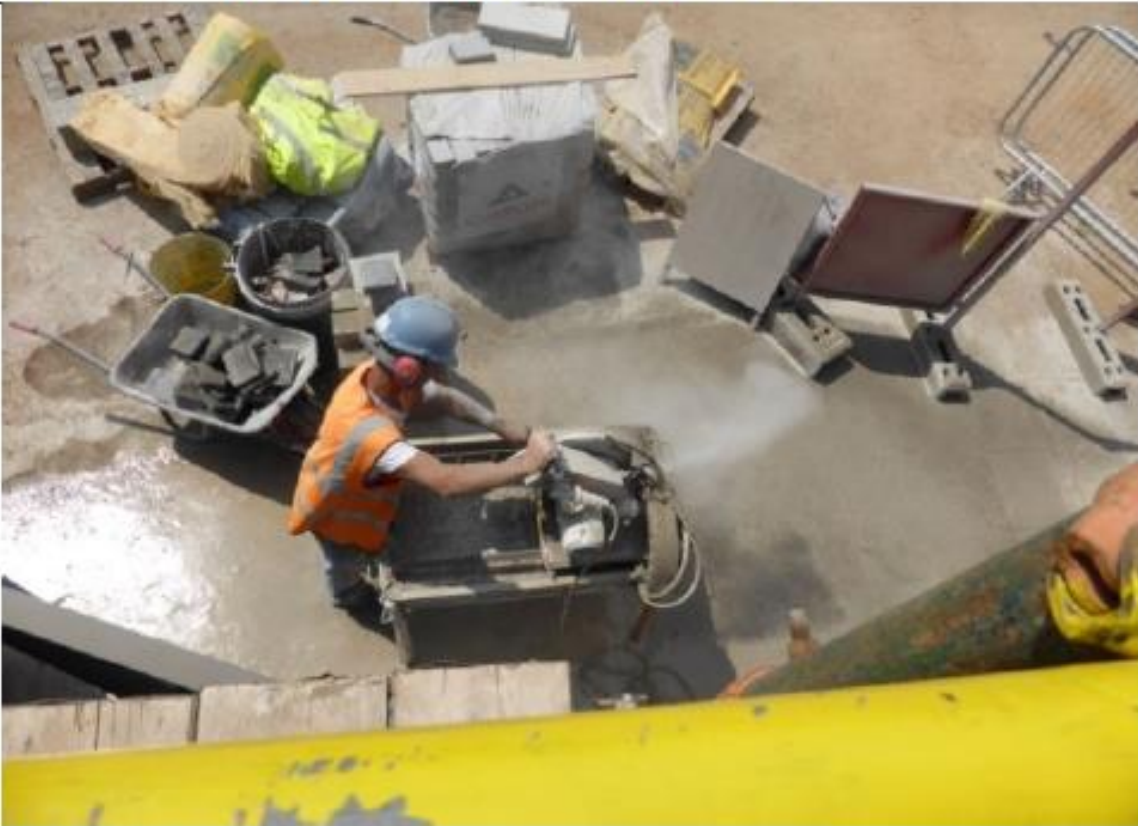
Poor Practice – No/insufficient water suppression and lack of RPE (HSE, GB)
