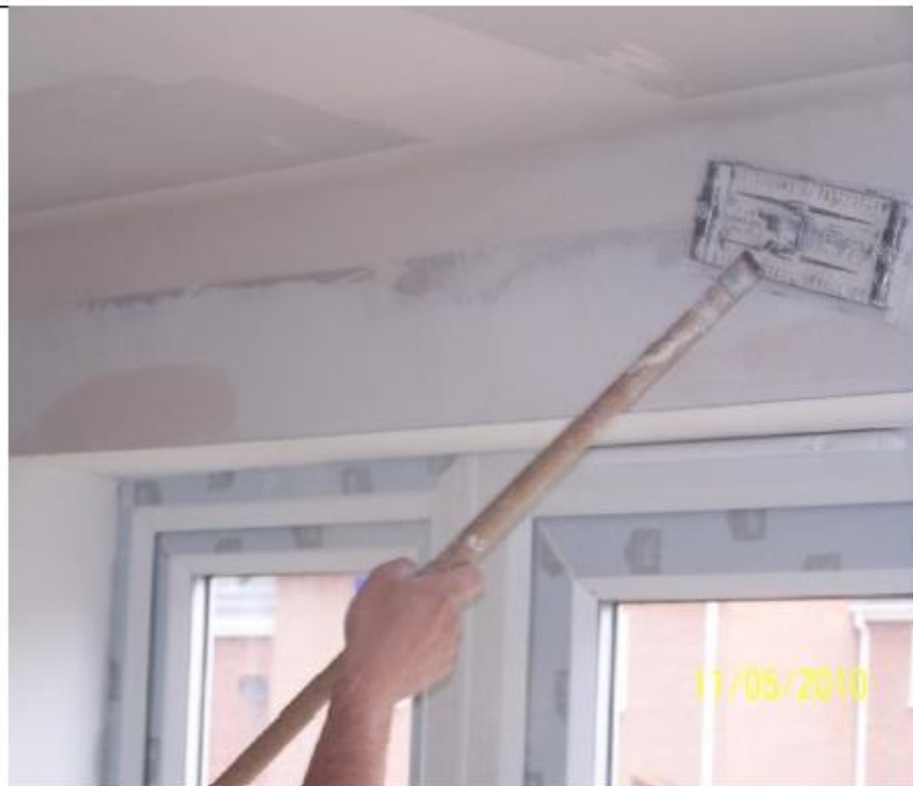
Poor Practice – Use of a pole sander without extraction (HSE, GB)
