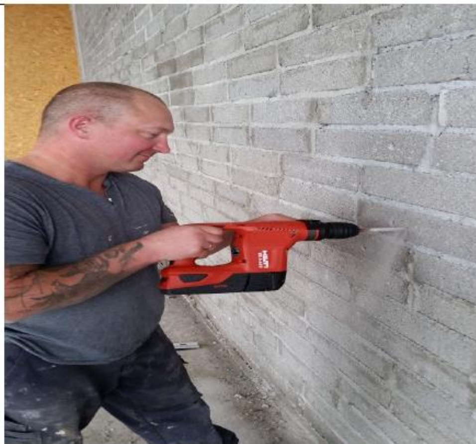
Poor practice – Using Hand-held drill with no on-tool extraction (David Flynn Ltd, IE)
