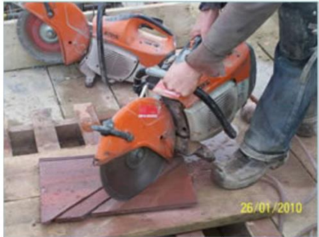
Good practice – Cutting roofing tiles with a tile cutter (National Federation of Roofing Contractors Ltd, GB)
