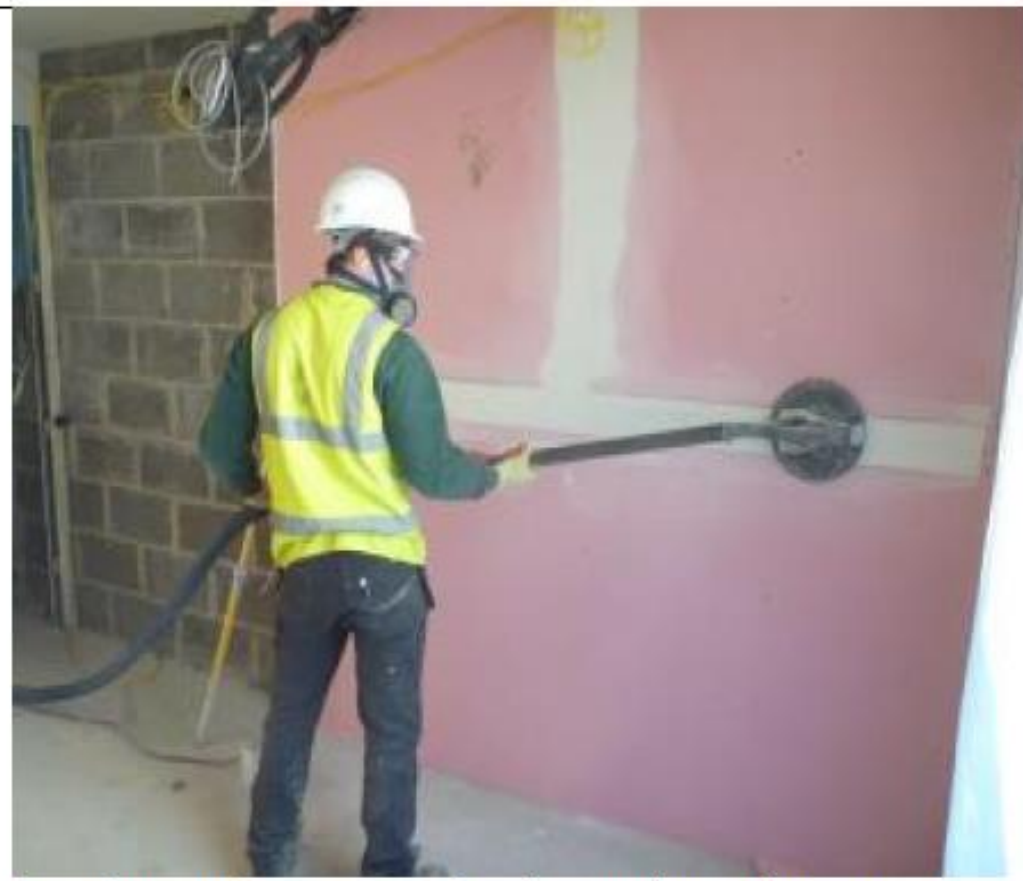
Good practice – Use of pole sander with extraction (HSE, GB)
